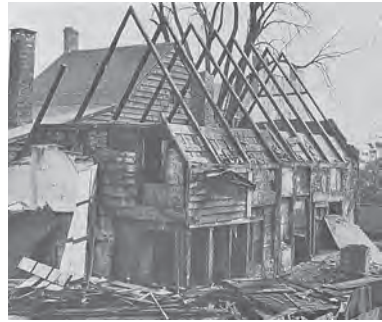
Figure 2 The razing of the Bradt house, Schenectady, in the late nineteenth century. The bent system of framing is clearly seen in this view
