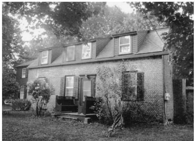
Figure 7. The David DeFrest house, c.1771. Photograph June 2004.
